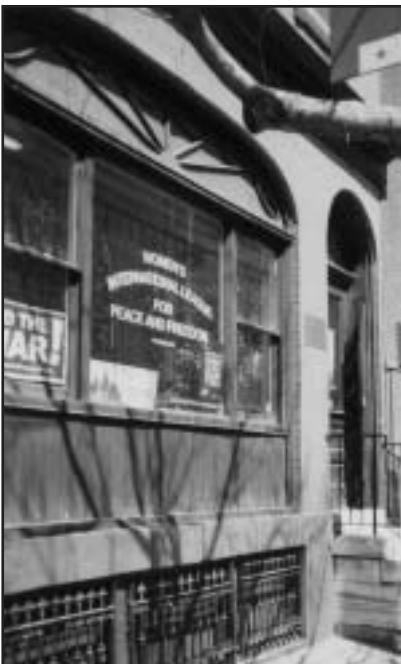
Building at 1213 Race
